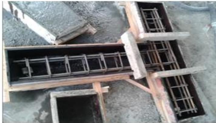
Figure 3. Steel cage placed inside the form work with proper cover
